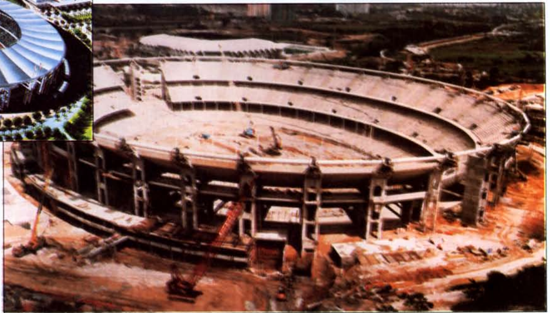
The Outdoor Stadium under construction at Bukit Jalil, Kuala Lumpur.
