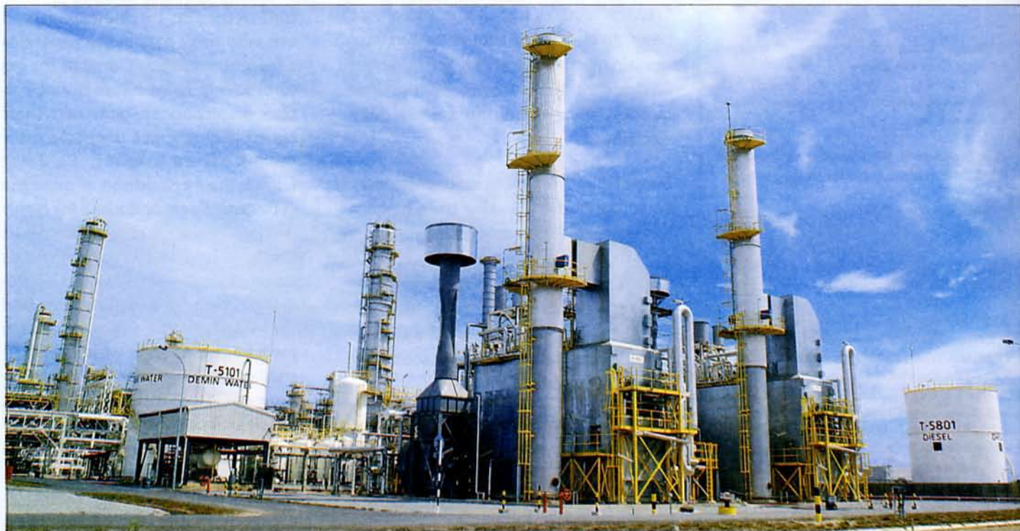
Crude Distillation Unit under the first phase of the Melaka refinery
