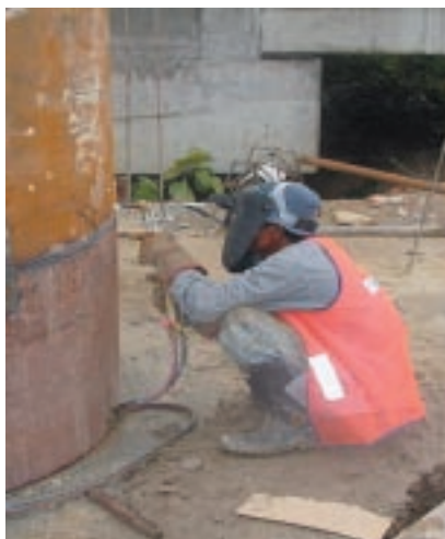
Welding work with proper personnel equipment
