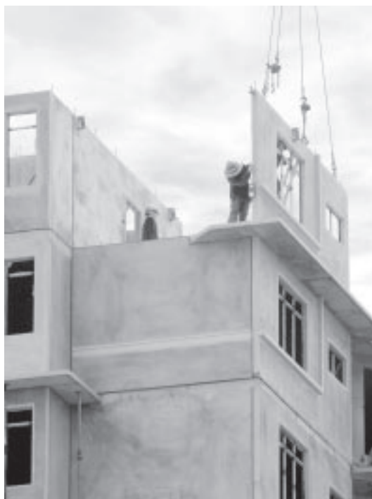
Installation of Precast Concrete Wall: Manpower – Critical Success Factor
