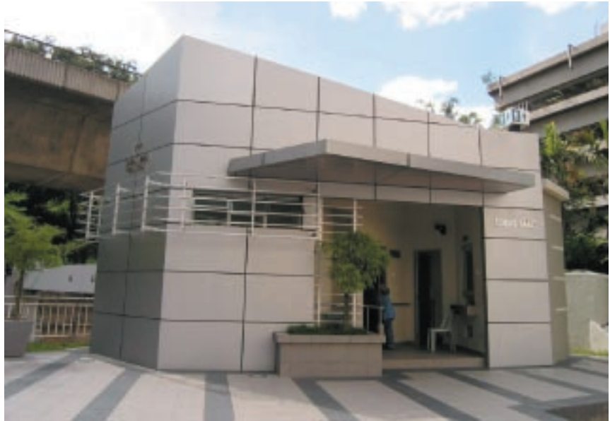
Street Toilet, Architect Department, City Hall Kuala Lumpur
